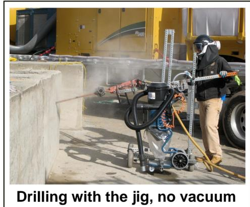
Drilling with the jig, no vacuum
