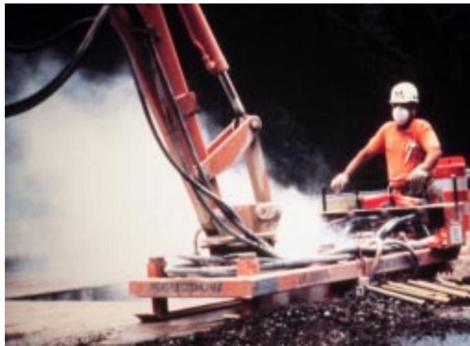
Construction worker exposure to silica dust during interstate highway repair.
