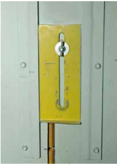
figure 5. Deflector slide (yellow) to prevent air from nozzles blowing into the face of shorter workers.
